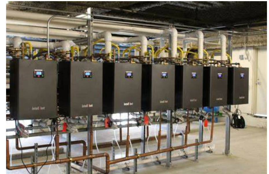
High Efficiency Gas-Fired Tankless
