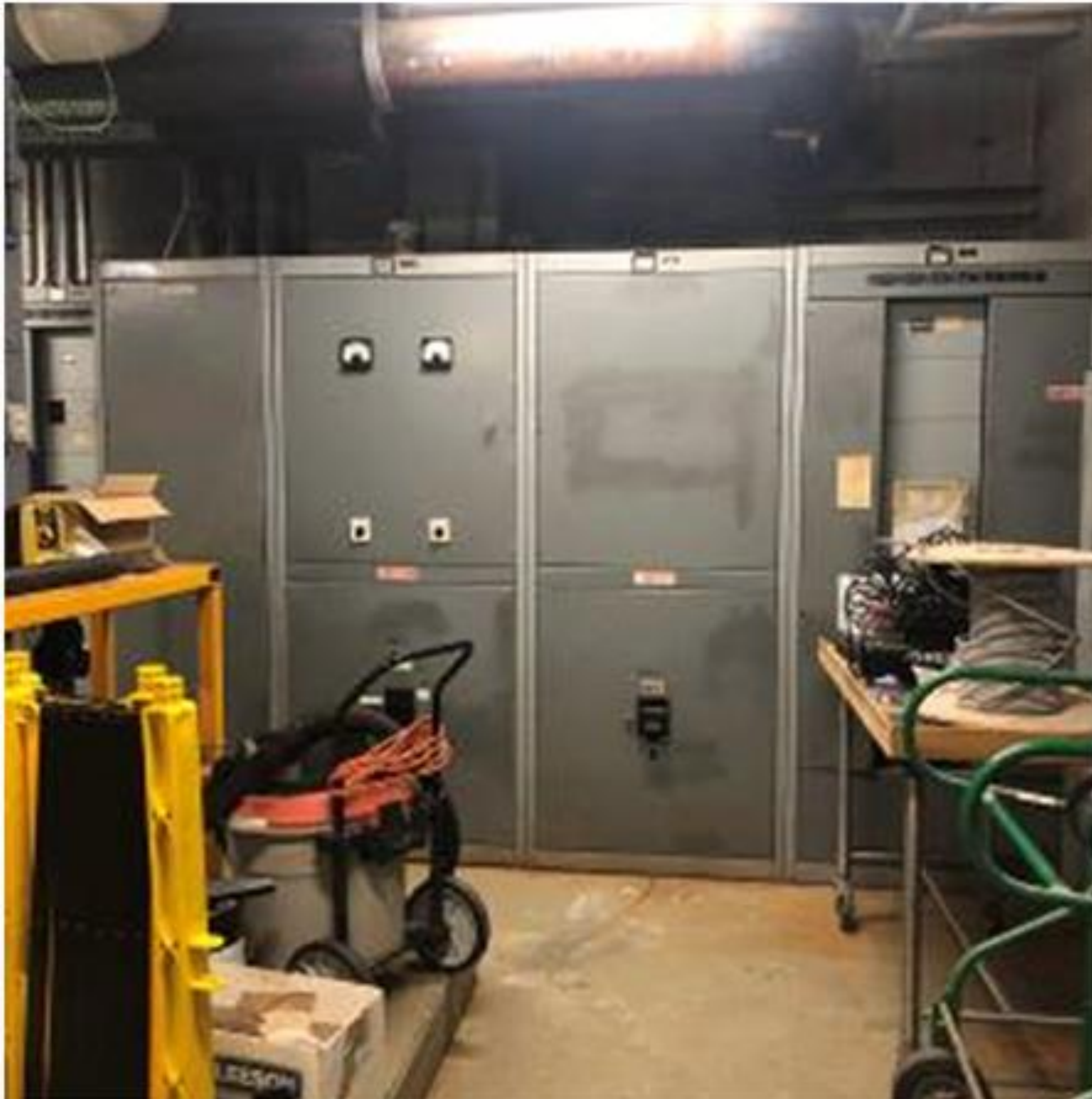
Electrical Switchgear
